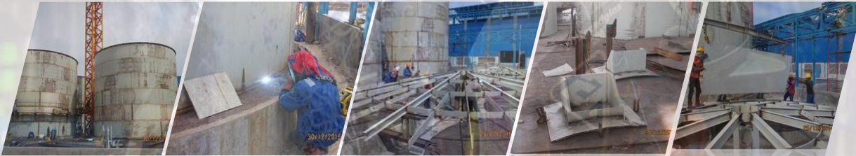
FABRICATION AND INSTALL STORAGE TANK CAP 1500KL
