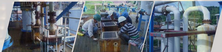
PIPE, SEALLING SYSTEMS, PARTS AND INSTRUMENT INSTALLATION
