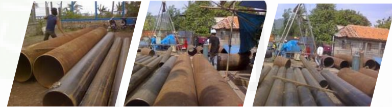
FABRICATION FOR GAS PIPELINE
